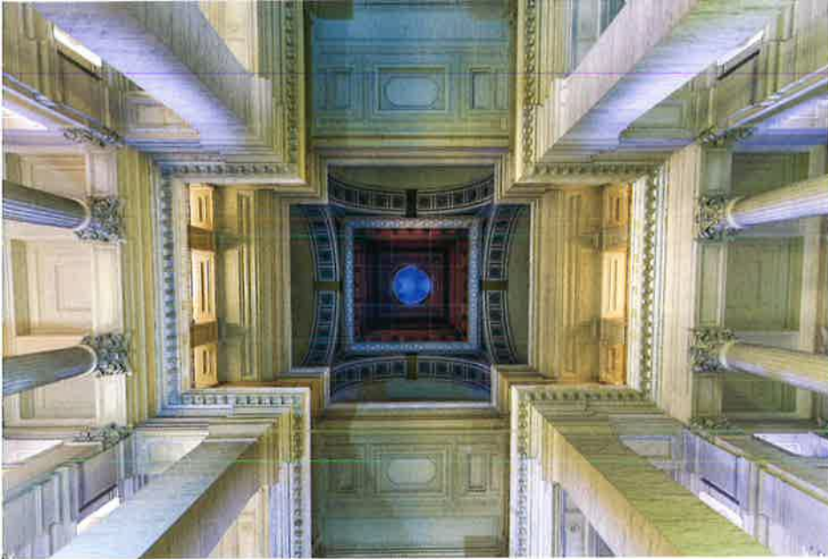
The ceiling above the portico
