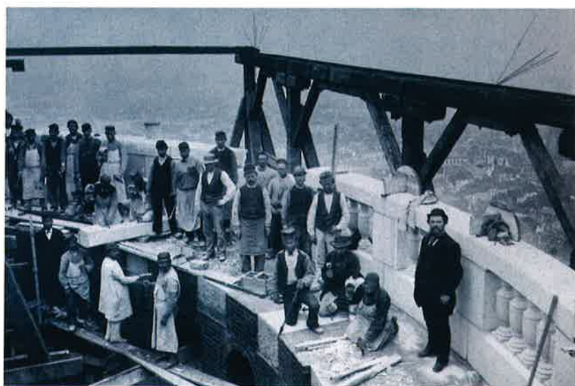
Workers building the dome
